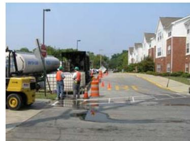
The pilot test confirmed reagent distribution and *in situ* zinc concentration reductions. The full-scale PRB application included a total of 45,000 gallons of slurry injected at 63 locations over 4 weeks. Within two years the zinc concentrations in the creek met the 2 mg/L remediation goal, and the site achieved regulatory closure.
